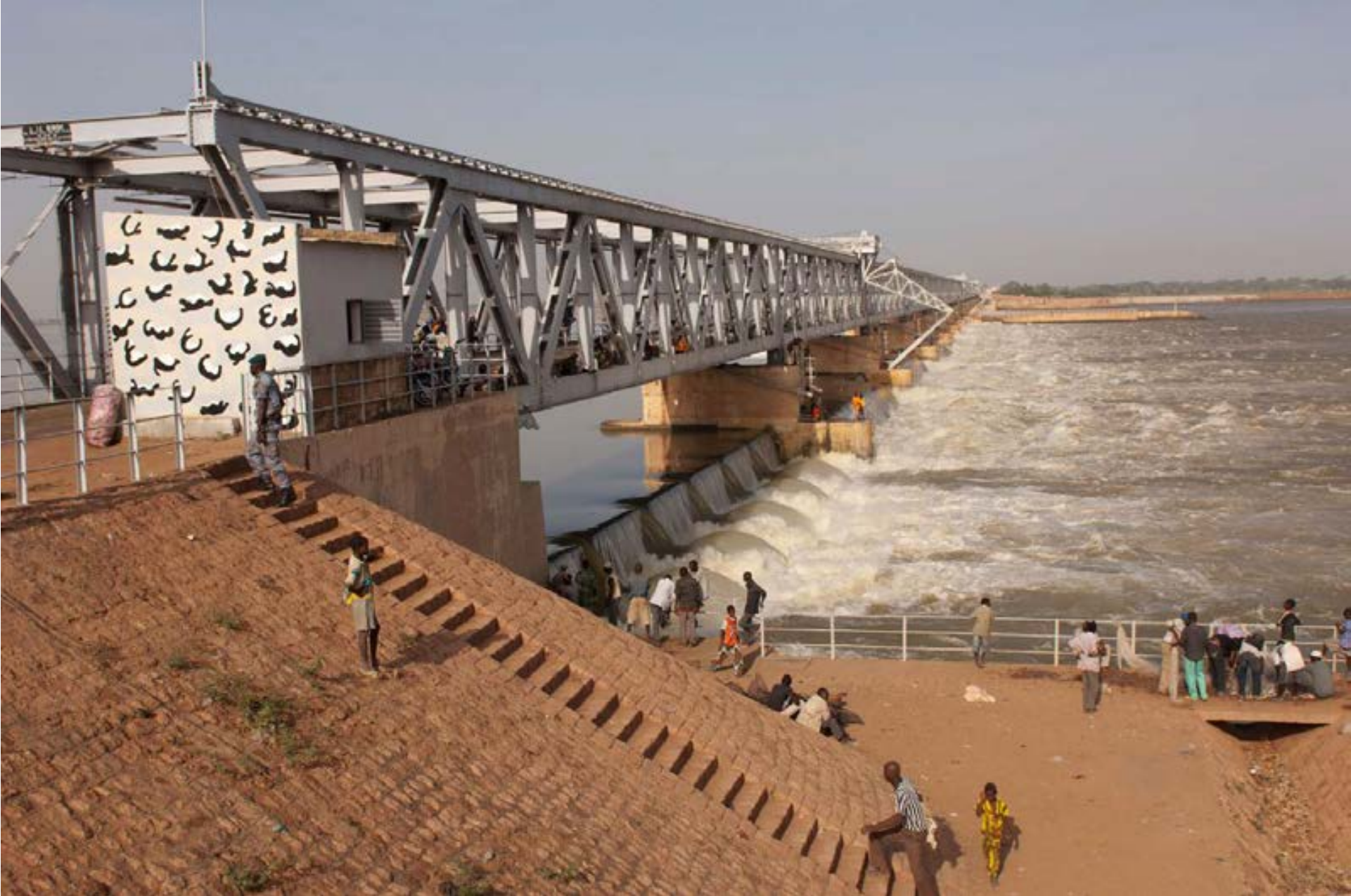
Mali's Markala dam (Image: Bert de Ruiter / Alamy), https://chinadialogue.net/en/nature/is-china-edging-away-from-a-massive-dam-on-the-river-niger/
