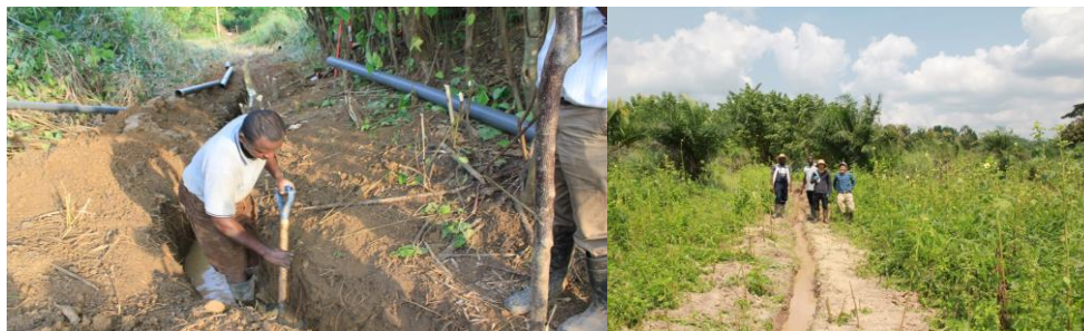
Restoration measure to connect spring water and sawah by irrigation canal and syphon pipes at Adugyama, Mr. Tawiah's site, August 2011
