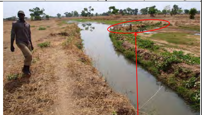
Photo 44: Nupe's traditional intake weirs and irrigation canals in the Pategi / Lafiagi region on the opposite bank of Bida, across the Niger River. This area is also used by Nupe people for rice cultivation and fishing. Weir using woods, grass, soils, and sand bags
