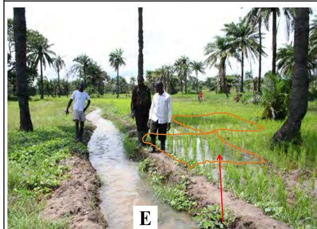
Photo 57E: Nupe's gravitational irrigation system with micro-rudimentary Sawah plots , Bida, Central Nigeria (September 2010).
