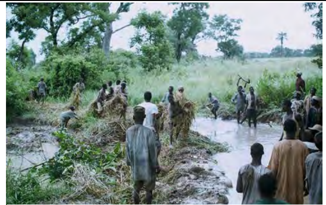
Photo 30: Farmers repair irrigation canals destroyed by the passage of large numbers of nomadic cattle and surface runoff from upland. The photograph was taken at location ③ in Figure 2.
