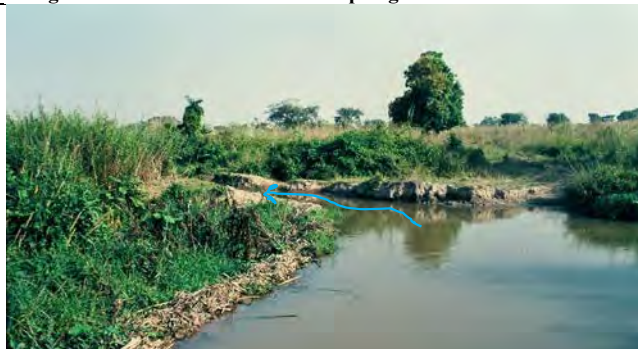
Photo 43: Construction of weir by Nupe farmers, using woods, grass, soils, and sand bags in Bida area, which is effective mainly in the dry season. In the rainy season, the weir is damaged, but the system can work as interceptor canal irrigation. This is one of the biggest one constructed on the Musa river, East of Bida. The blue arrow indicates irrigation canal. This photo was taken in February 1987
