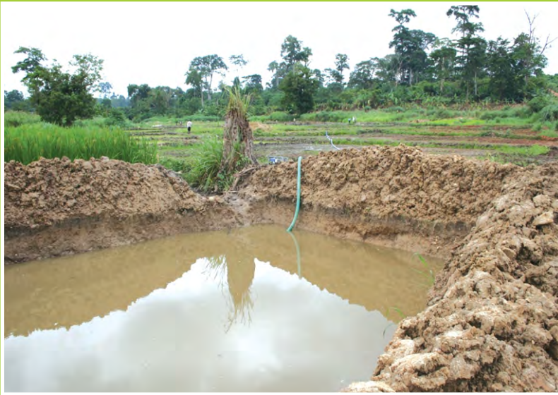
Small pond may be constructed by farmers, when necessary for water to irrigate (e. g. Kodadwen, Ghana)
