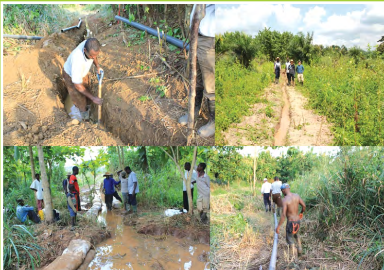
Restoration measure to connect spring water and Sawah by irrigation canal and syphon pipes at Adugyama, Mr. Tawiah's site. August 2011. This site was destroyed by IVRDP through poor knowledge of Sawah system development.
