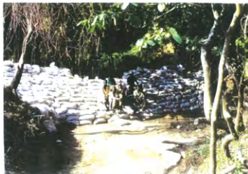
Photo. 3-26. Dyke was covered with sand bags after compaction of permeable layer
