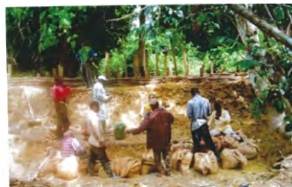
Photo. 3-23. Excavation of river bottom and jute bags
