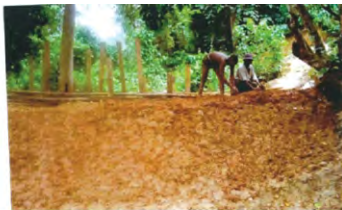
Photo. 3-25. Compaction to create impermeable layer on the front of dyke, March 2000
