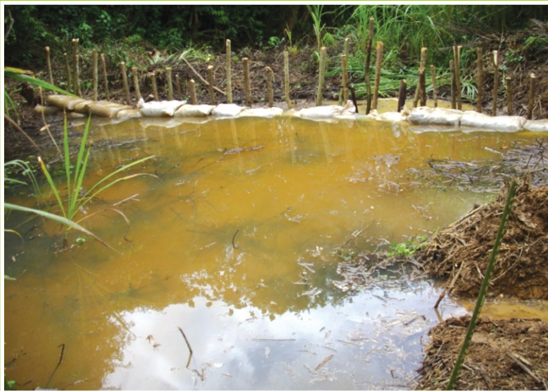
Water harvesting structure (weir) using local materials is ready and water impounded for diversion to rice fields
