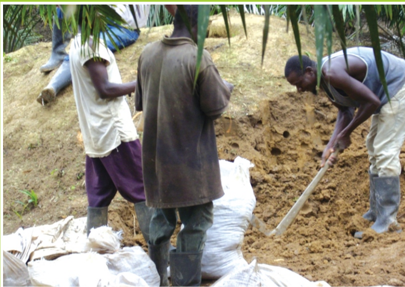
Empty polyethelene sacks may be filled with soil from adjacent high land/hill, preferably closed to source
