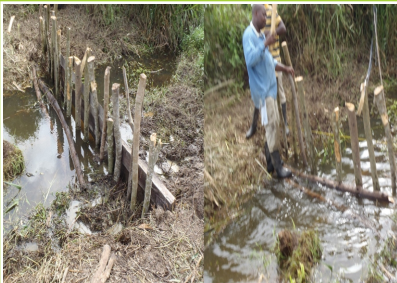
Wooden poles, harvested on or around the fields should be firmly fixed on the ground across the water sources (eg. Stream)
