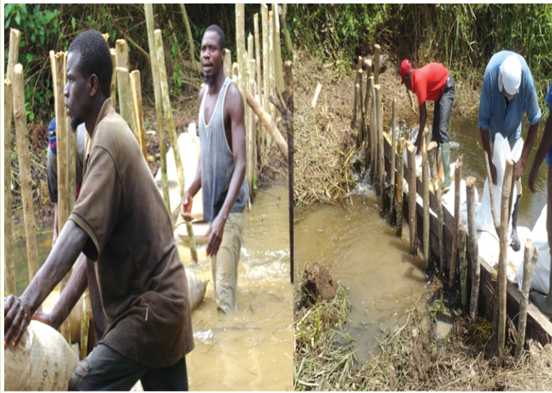
Sand bags are then lined infront of wooden poles that have been firmly put into he ground
