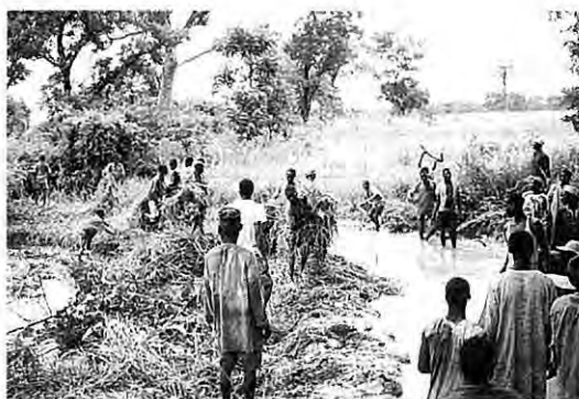
Photo 6-14 Repair work for the destroyed bank of the irrigation canal
