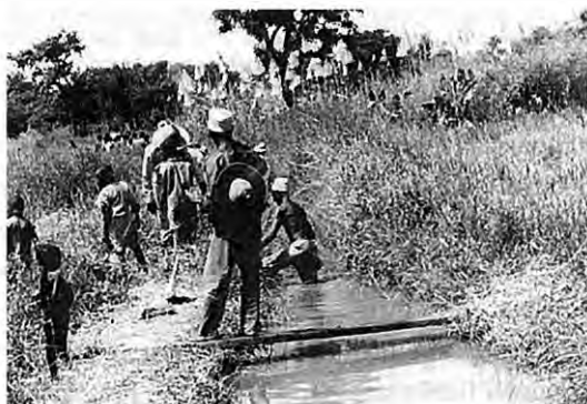
Photo 6-11 Maintenance work of irrigation canal by the joint efforts of community members (August 1995)
