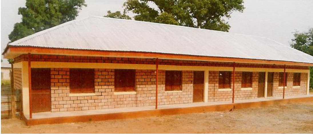
Figure 1: Shaba-Maliki, A block of Classrooms.
