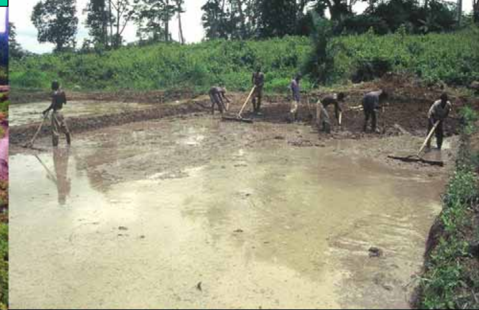
The leveling needs skilled & concerted works
