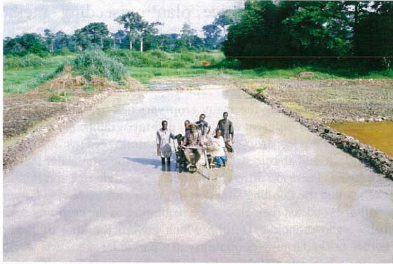
Photo 4-7 Just after the completion of leveling by power tiller
