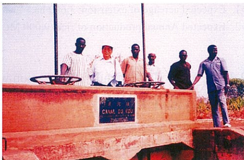
Fig.9-2. Irrigation water intake control gate at Kou built by Taiwanese Mission. Fifteen-km long irrigation canal takes water through this gate to irrigate the newly reclaimed rice field of 1,260 ha at Kou, Burkina Faso. The author (second from left) posed with the farmers at the water gate.
