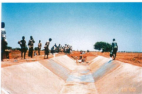
Fig.9-1. Construction of irrigation canal as a part of land reclamation project at Bagre, Burkina Faso.
