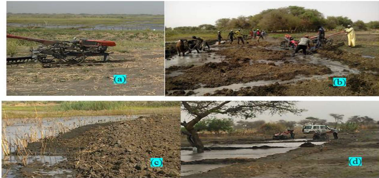
Fig. 7 a.) pre-intervention; b.) during poldering; c.) soil and water interface; and d.) levelled basins ready for rice seedling transplant
