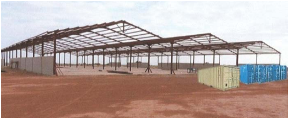
Figure 67: Export Crop Handling, Preservation and Conditioning Center, Ambursa, Kebbi State (Ongoing)
