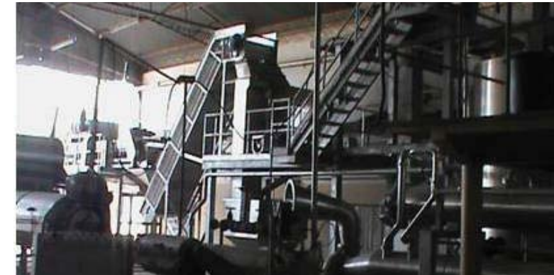
Figure 50: An orange juice processing facility
