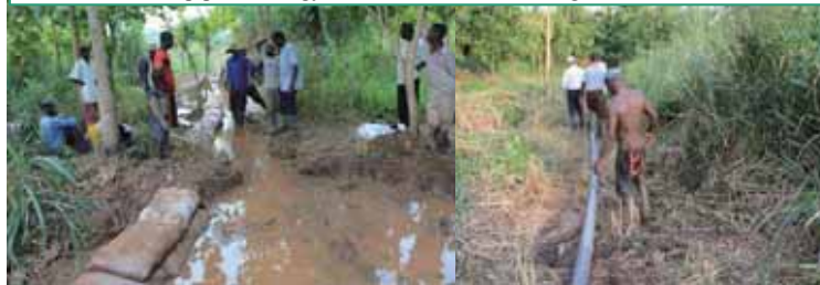
Sand bag weir by farmers and SRI Sawah team, Aug.2009, Nsutem, Ghana
